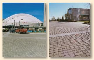
Adjacent to the Toronto SkyDome and the CNTower inToronto, this fire station uses PICP to reduce runoff pollutants entering nearby Lake Ontario.
