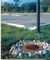
Three layers of open graded base enabled filtering and drainage while providing a stable structure during construction.
