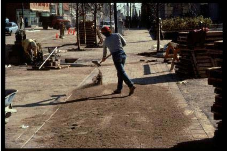
Figure VI: Joint Sand is spread on the pavement. Also of note is the soldier course used on pedestrian areas adjacent to the cast-in-place concrete edge restraint.
