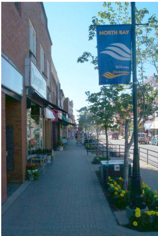
Figure IX: The back of sidewalk cast-in-place edge restraint at the building interface was beneficial both from a uniform visual appearance and with offering an easy way to set grades for the back of sidewalk
